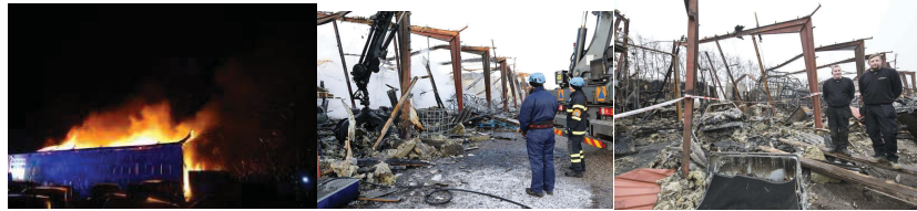
Picture 3 The warehouse with all the spare parts burned down.
